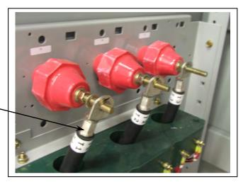
(18) Remove four thread former screws holding motor connection terminal assembly into the cell. Carefully move this assembly up to the top cell and lay onto the main contactor rail area.
