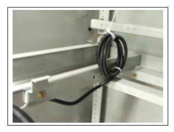
(17) Remove load cables from insulators. Pull cables through the CT and remove from the cell.
