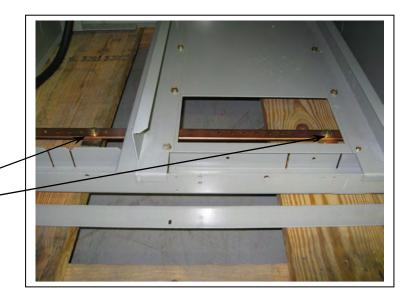
(6) Remove motor connection insulators and CT and flip where motor connections are on bottom.
