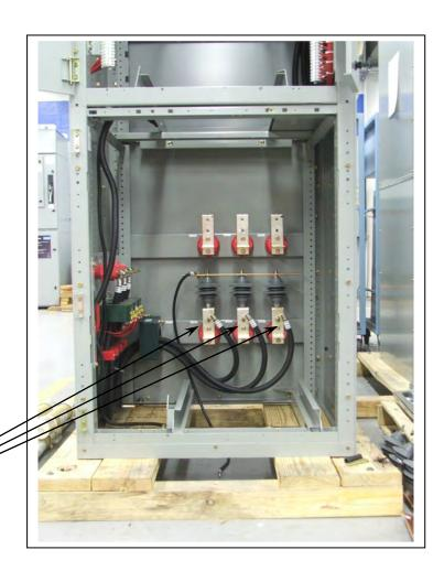
(15) Remove two bolts holding Ground Fault CT. Remove low voltage wires and keep GFCT assembly for reinstallation.
