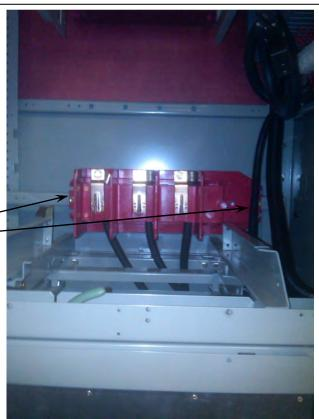
Replace screws to hold assembly into cell
