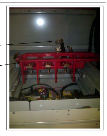
(13) Attach glasspoly part to cell. Make sure to place flat glasspoly barrier in back of part before attachment to cell.
