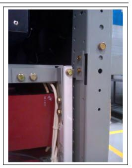
(20) Attach low voltage plug to RVSS truck. Attach fiber optic cables to main circuit board in low voltage bucket. Be careful not to bend fiber optic cables.
