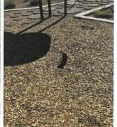
Lady Bug Spring Toy is missing handhold. Bolts missing from swing cross bar mount. Swings missing completely. Paint has chipped off of swing post. Spring toy is completely missing exposing a large metal piece from the woodchips. Recommend immediate removal of the spring tov bracket. High probability of injury.
