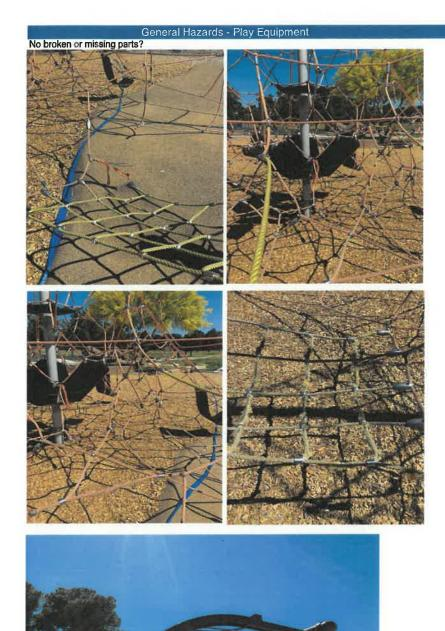
Wirte Rope Climbers have several locations where ropes have become broken and internal wiring is exposed. Immediate removal of damaged ropes is recommended. Track rider is inoperable and should be repaired or replaced. Track rider has parts coming apart that could have possible cut hazards.
